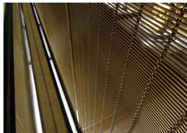
View between the railing and screen: Glare is reduced by honeycombed louvers (The line of light showing on the left is a reflection on the glass railing.)
