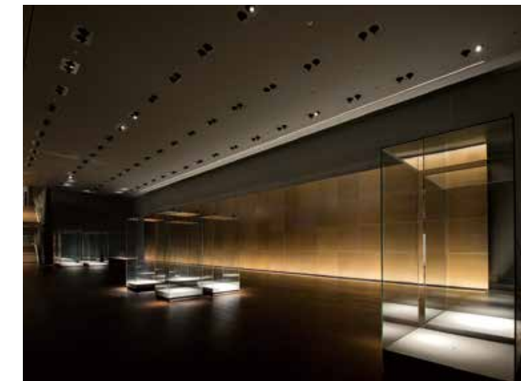
Lighting fixtures for front lighting in the sculpture gallery are hidden under the floor and in the ceiling.
