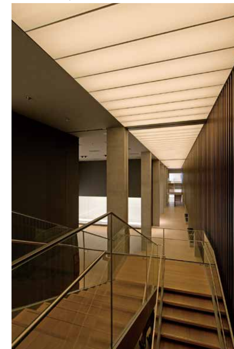
Lighting for the passageway connecting the 2nd floor galleries: The continuous luminous ceiling is uniformly illuminated using a minimal number of lamps.
